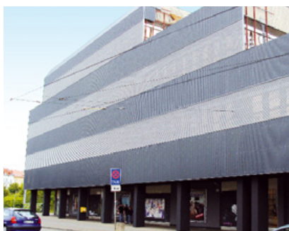
Karstadt Halle - Germany, Aluform sinusoidal profile 18/76 perforated and non-perforated
