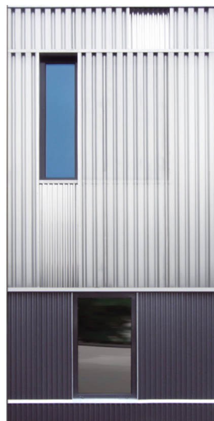
Station Vienna West - Austria Aluform trapezoidal profile 45/150 blank smooth, perforated
