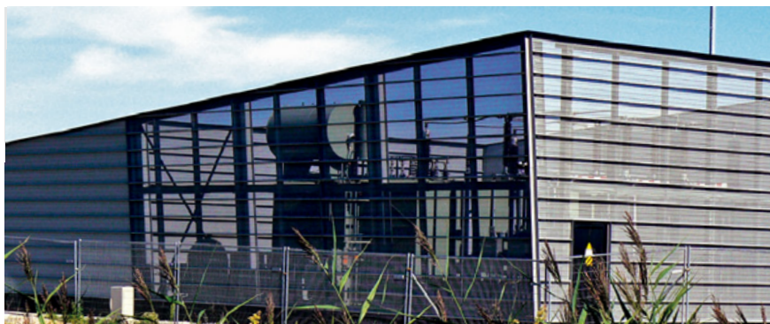
Erdgasbuffering Zuiderwending - Netherlands, Aluform standing seam profile 64/400 perforated
