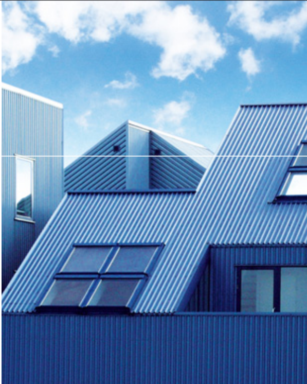
Floating apartments, Ijburg Trapezoidal profile, Aluform 29/124
