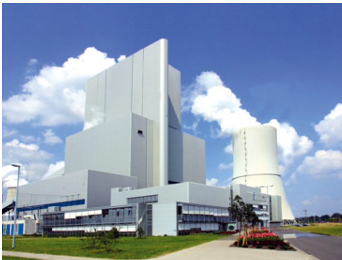
Power station, Boxberg Trapezoidal profile, Aluform 45/150
