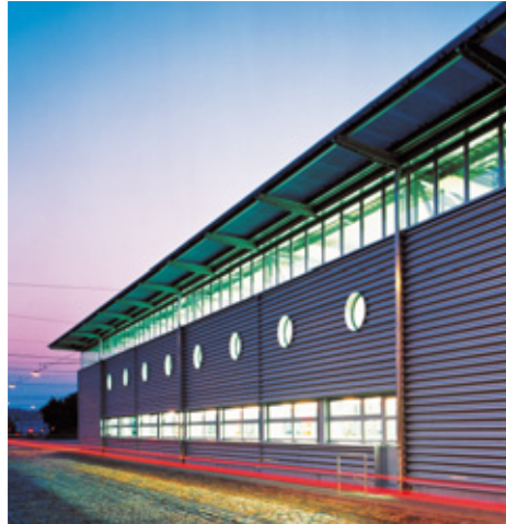
Industrial hall Sinusoidal profile, Aluform 18/76
