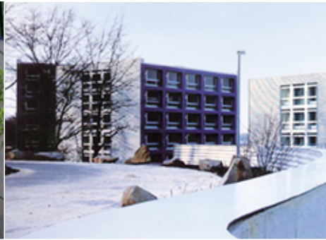
Hall of residence, Wuppertal Sinusoidal profile, Aluform 18/76
